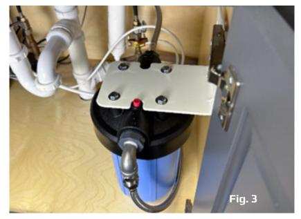
**Note:** Some faucet manufacturers have integrated supply lines on their faucets from the factories. These are compatible with the discharge fitting on the housing. Once the unit has been installed completely, open the cold side of the faucet, slowly turn on the cold-water supply and allow the water to flow from the kitchen faucet for about 10 minutes. This is to rinse the media and to purge any air out of the cartridge. Once the time is up, turn the cold water off and check for any leaks.
