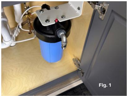
Attach the appropriate length supply line to the cold-water supply stop and connect the other end to the  $\frac{1}{2}$ " stainless nipple on the front side of the unit. This is your cold-water inlet. (See Fig. 2)
