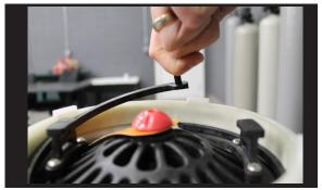
Remove snap ring and tank top from tank.
