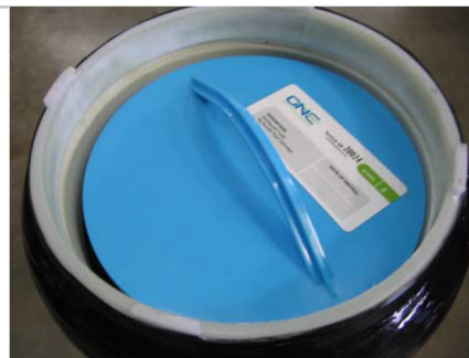
A filter this high is not installed properly.
